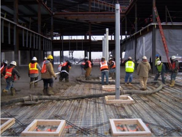
WELDED WIRE FABRIC: CLUTTERED DECK WITH EXTENSIVE TRIP HAZARDS, MESH OUT OF POSITION RESTING ON TOP OF DECK
